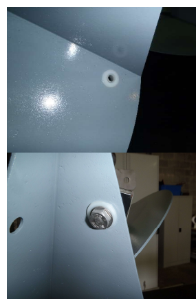
Figure 35 plastic insulation between different metals
